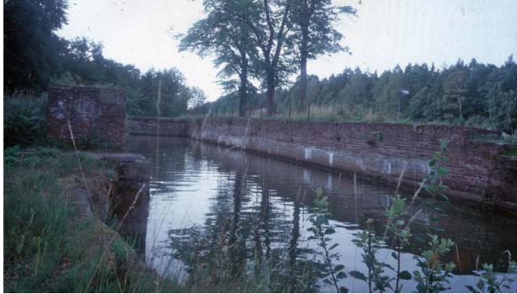
Fig. 1 Gustaf's Locks at Brinkebergskulle in the Göta River, constructed 1772-78 with an alum shale mortar from the cement factory at Brinkebergskulle. Photo: Sölve Johansson 1989.
