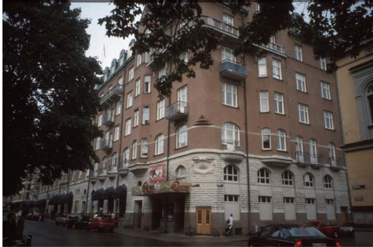
Fig. 2 Örebro render at domestic house in central Örebro. The house was built 1912-13 with a red render based on burnt alum shale from Latorp near Garphyttan. Photo: Sölve Johansson 2002.
