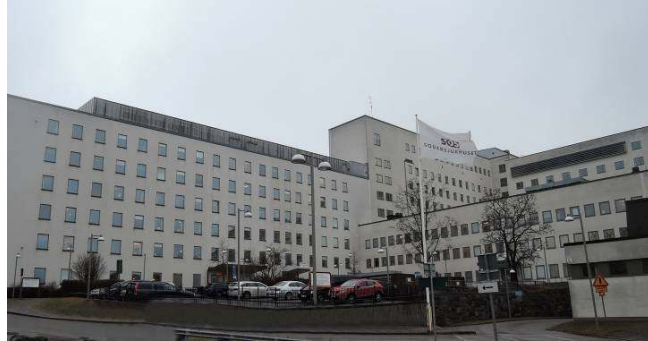
Fig. 3 The southern general hospital in Stockholm
